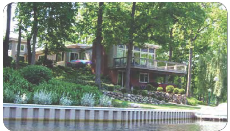
Above: Even though this property has a seawall instead of a natural shoreline (see tip #3), the homeowner is trapping runoff with a vegetated buffer. Photo by Victor Banta Photography
