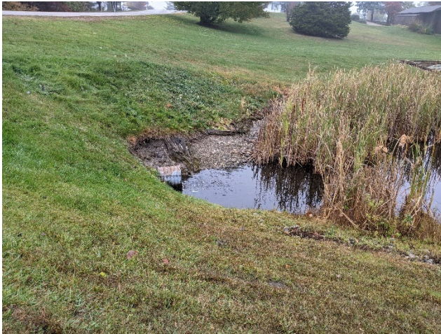
Outlet culvert at Critical Source Area 2
