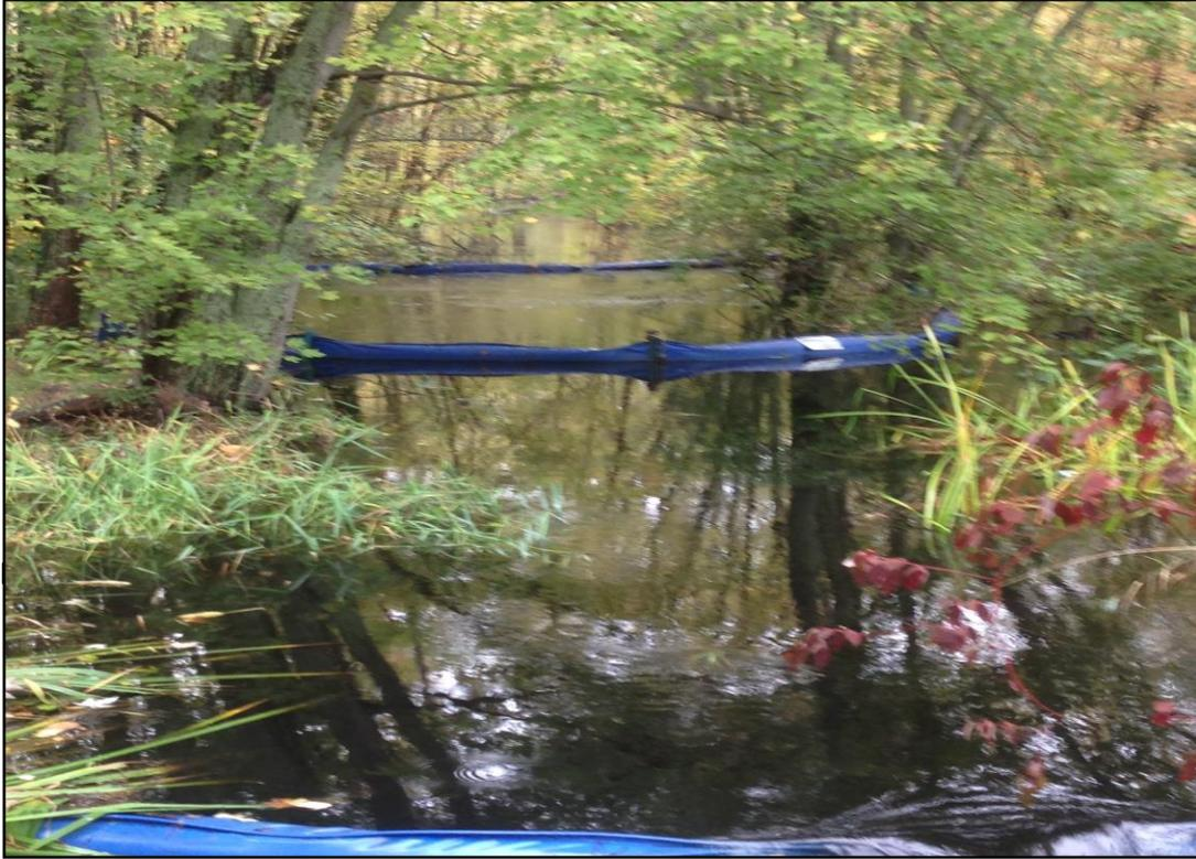
Figure 30. Example of a tributary/drain filter.
