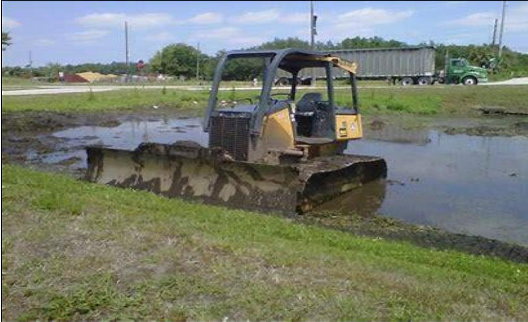
**Figure 33. Example of storm water maintenance (sediment trap removal).**
