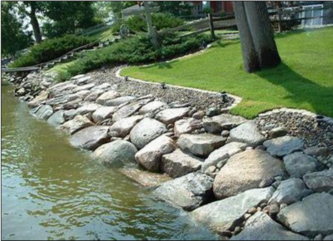
Figure 28. Example of armored protection/riprap.
